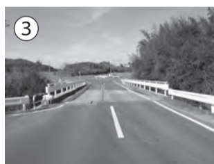
③ 萩野橋橋梁修繕事業(田茂町)
